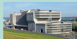
Waste incineration power facility in Perlen, canton of Lucerne (Switzerland)
