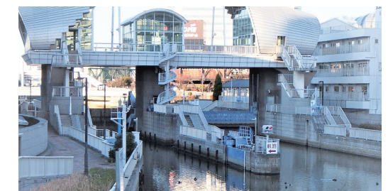
Dotonbori River Water Gate (Osaka City)
