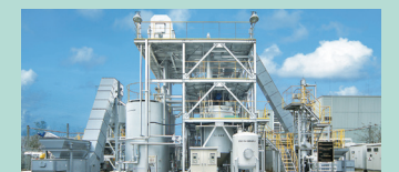
Bioethanol production demonstration facility (Kyoto City, Kyoto Prefecture)
