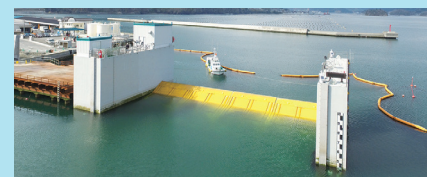
Overall view of seabed-type movable flap-gate (Iwate Prefecture)
