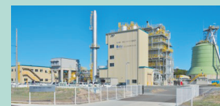
Miyanosato Woody Biomass Power Generation Plant (Hitachiota City, Ibaraki Prefecture)
