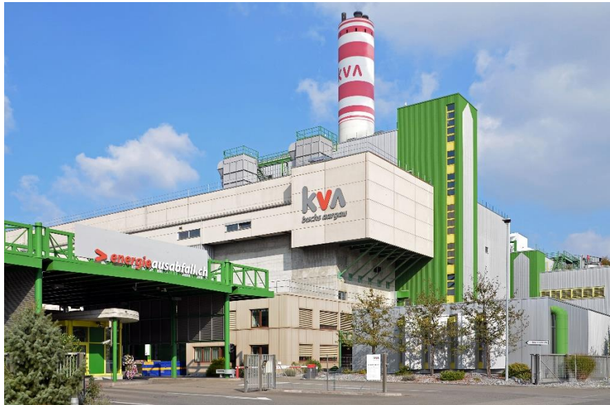
The EfW plant to be used in the project
