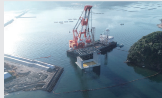
Seabed-type Flap-Gate for Hyogo Prefecture
