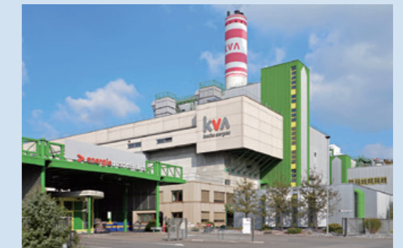
EfW plant used for this project
