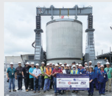
Concrete casks in Three Mile Island in the United States *U.S. subsidiary NAC International was in charge of engineering, while the Company was in charge of canister manufacturing
