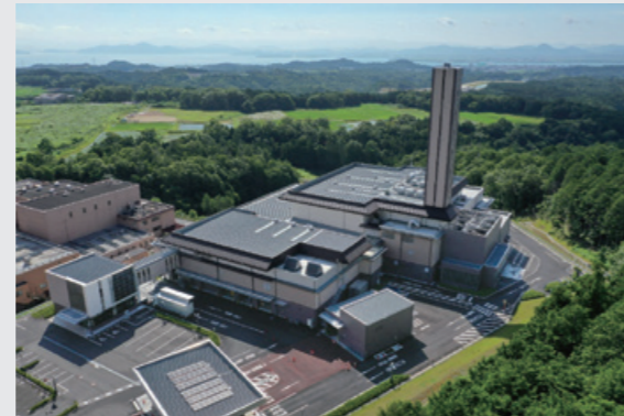
Waste treatment facility (North Clean Center) for Otsu City
