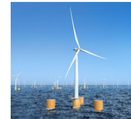
Offshore Wind Power
