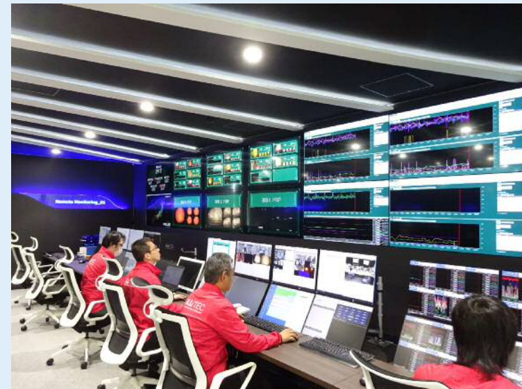
Remote monitoring and operational support area
