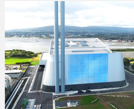
Dublin Waste-to-Energy Plant
